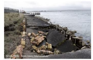
EXISTING DAMAGED SEA WALL
